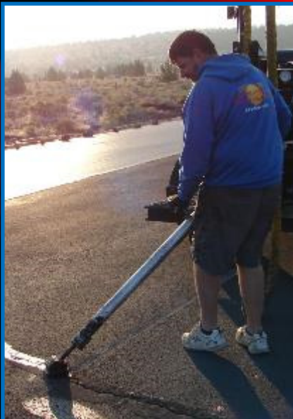
Lots of Crack Sealant
